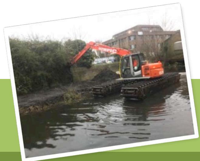
“a specialist amphibious excavator was used to overcome the deep water and poor access.”
